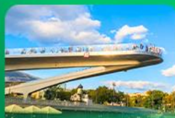
Floating Bridge Moscow
